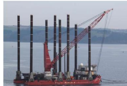
d) Jackup barge
